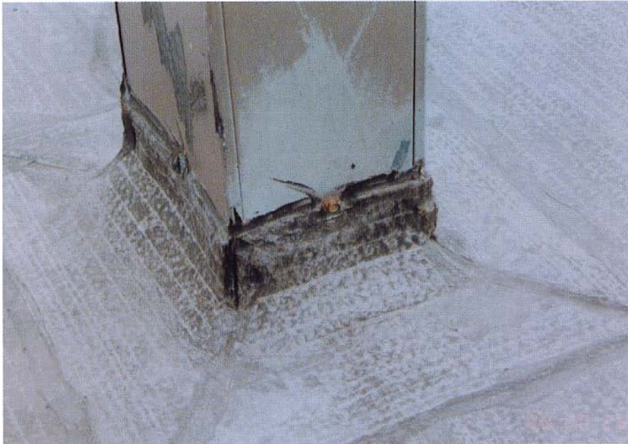
Photo 16: The roofing is welded outside the bushing and is in good shape after 10 years (from T2).
