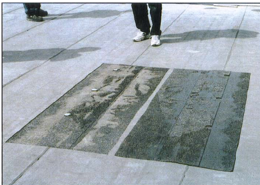
Photo 1: Sample taking. The roofing was mechanically fastened to the old roof. Underlayer was old asphalt roofing. The fasteners are placed close to the edge of the roofing (from T9).
