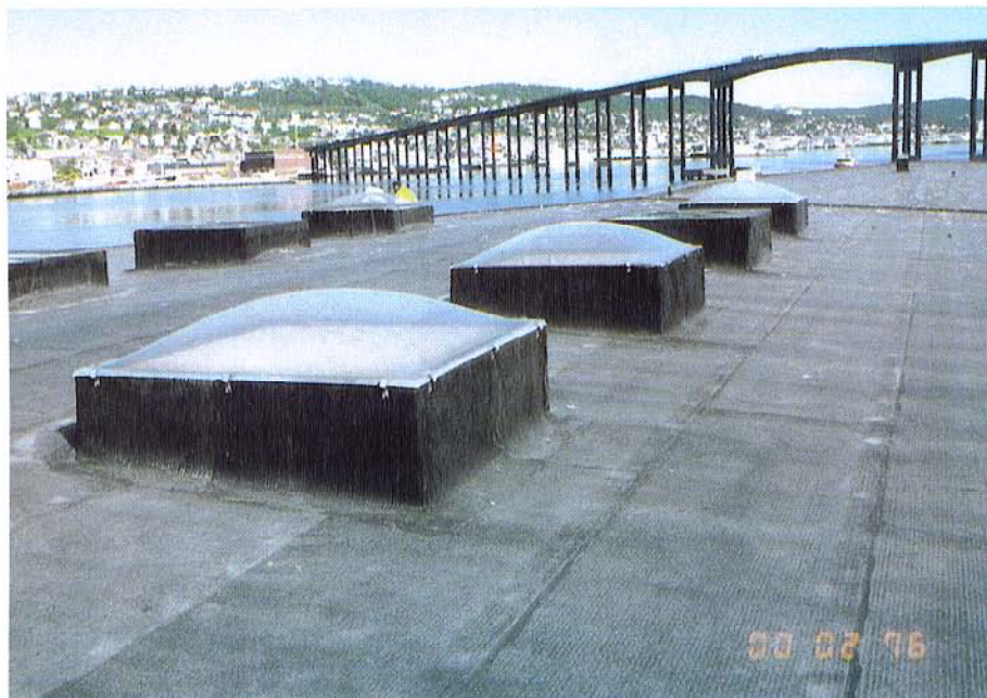
Photo 20: A large roof with a lot of sky-lights. Well done workmanship (from T14).
